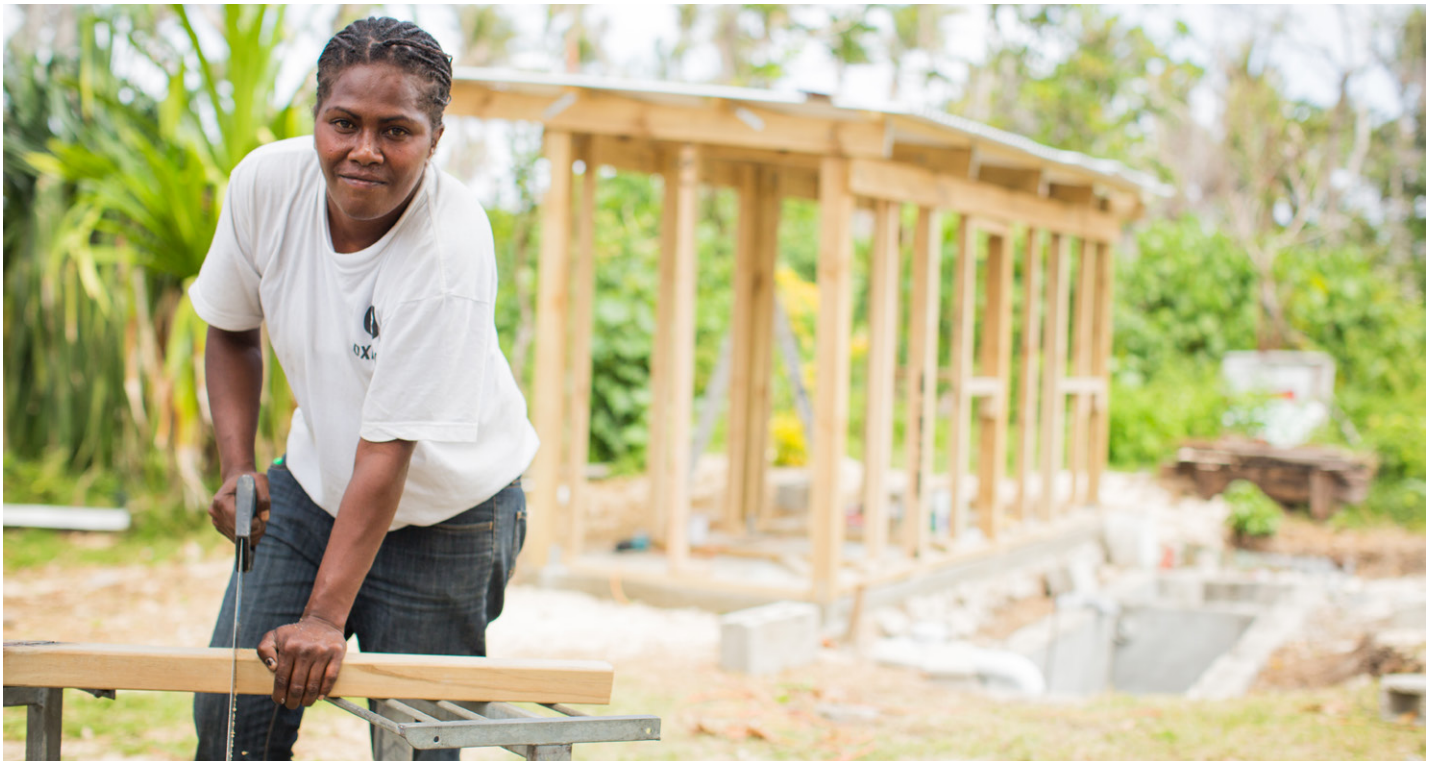
Eton, Vanuatu: Bryna Palmer is a Vanuatu Oxfam staff member on the WASH team. Bryna is breaking the gender moulds of her culture by working installing toilets in communities around Vanuatu. Photo: Arlene Bax/OxfamAUS.
